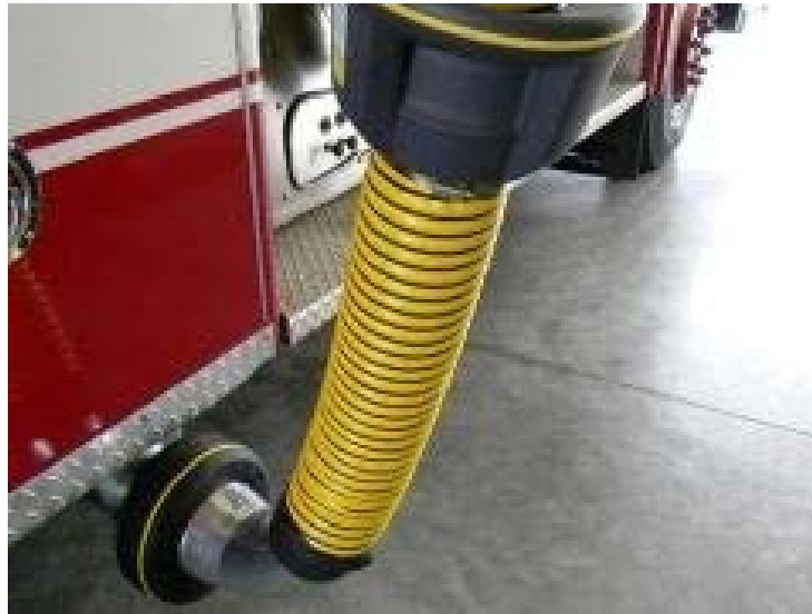
Figure 28. Source Capture Diesel Exhaust Extraction System
