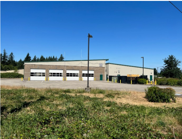
Station 91-Staffed Station 600 NE 267th Avenue, Camas, WA 98607
