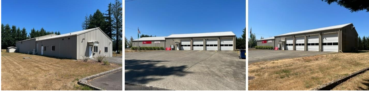
Figure 31. Station 94, 1808 SE 352nd Avenue, Washougal, WA 98671
